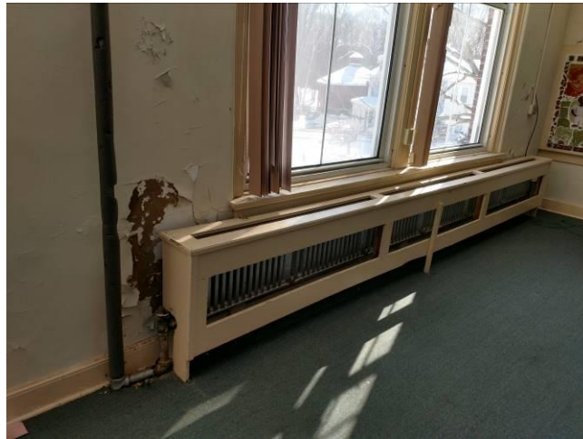
Cast Iron Radiator in Architectural Enclosure
