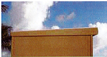
Sloped top for moisture runoff
