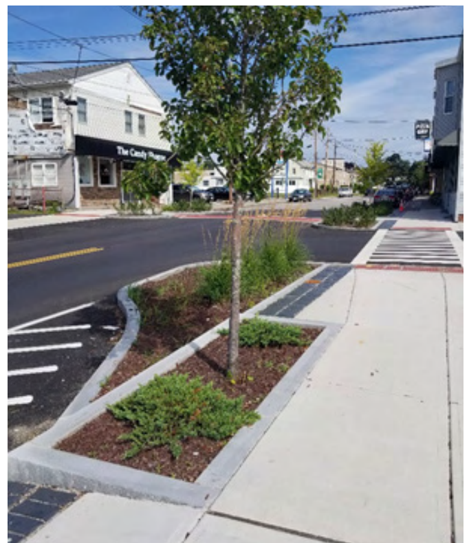
New sidewalks and bioretention features on Main Street. Photo credit: BerryDunn
