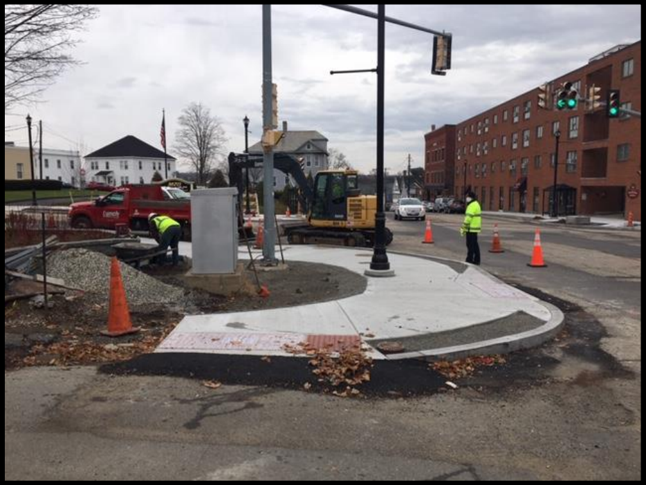
Intersection (Upper Common Side) Drainage Manhole (November 30)
