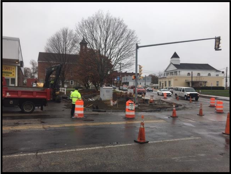
Intersection (Upper Common side) Curb Installation (November 13)
