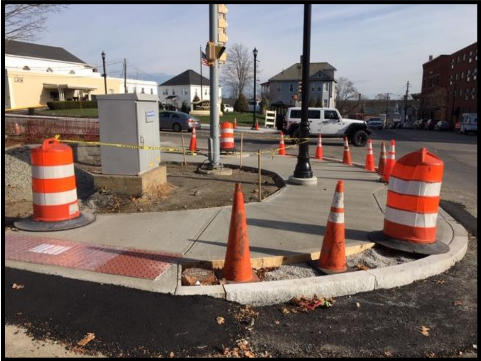
Intersection (Upper Common side) Sidewalk & Drainage Installation (November 20)
