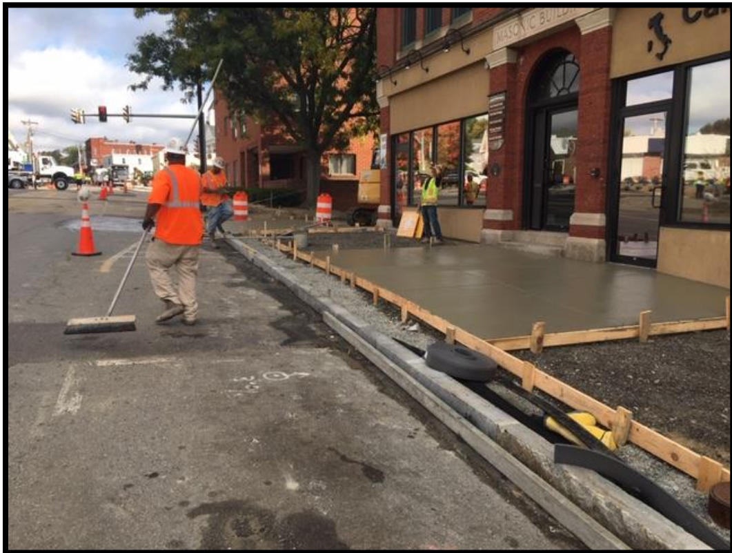
South Main Street (east side) Sidewalk Installation
