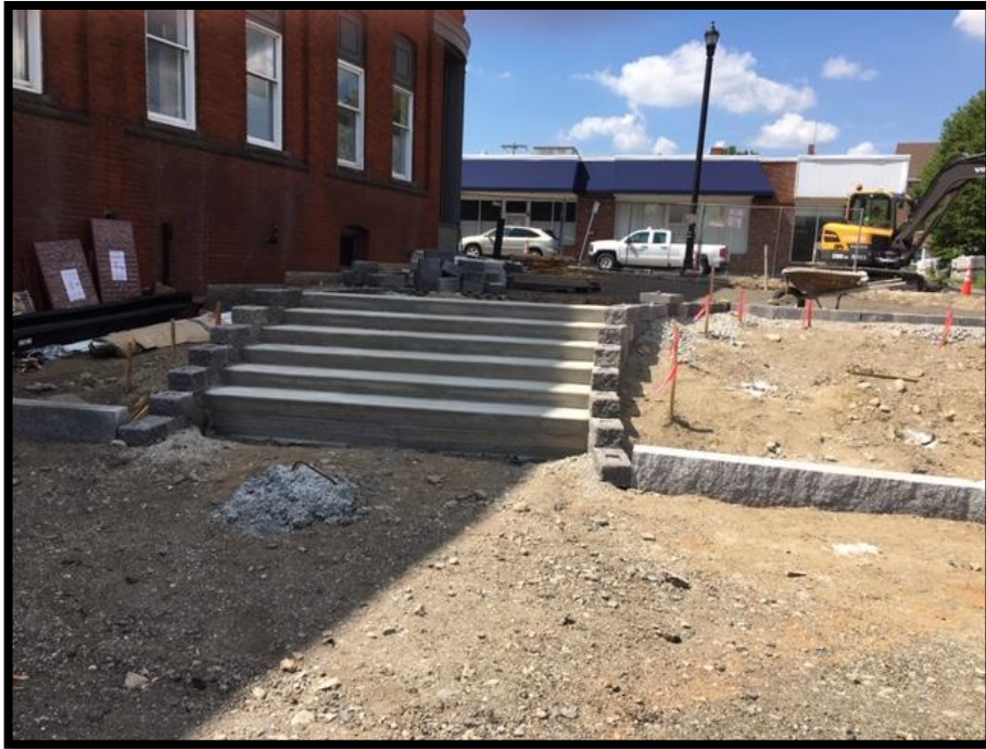
South Main Street – Lower Common Pedestrian Plaza/ Concrete Stair Installation (August 10)
