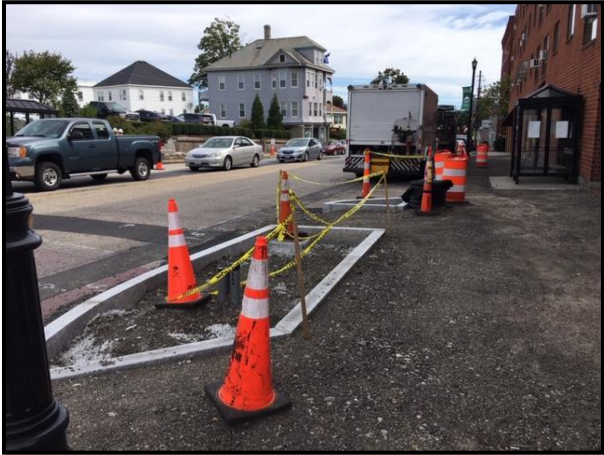
Elm Street (east) Sidewalk and Bump Out Installation, Curb Reset (August 26)
