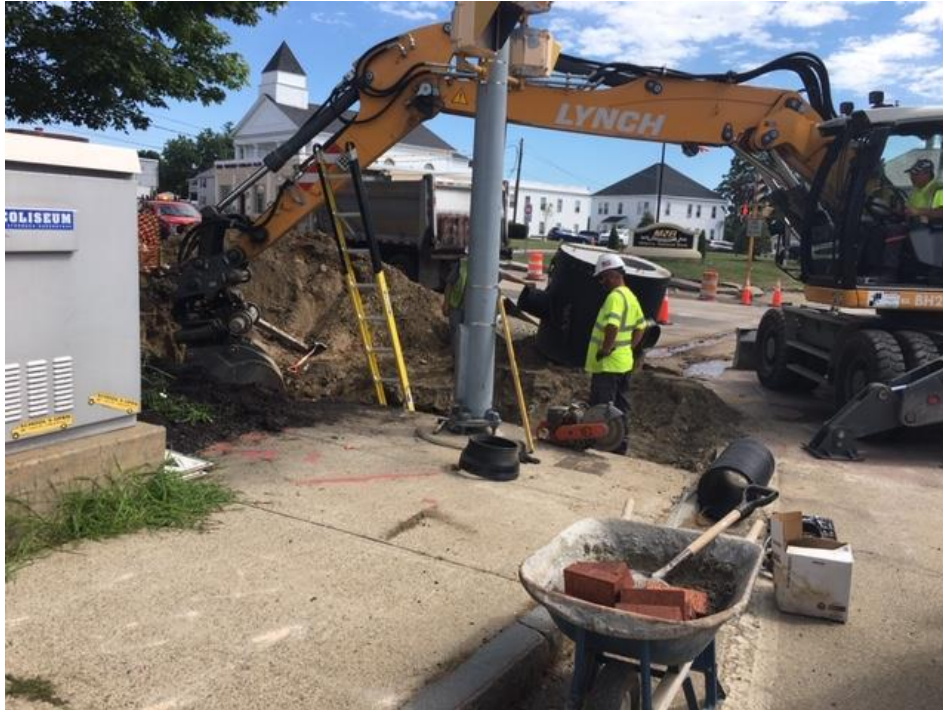
Main Street – Upper Common Pedestrian Plaza (catch basin installation)
