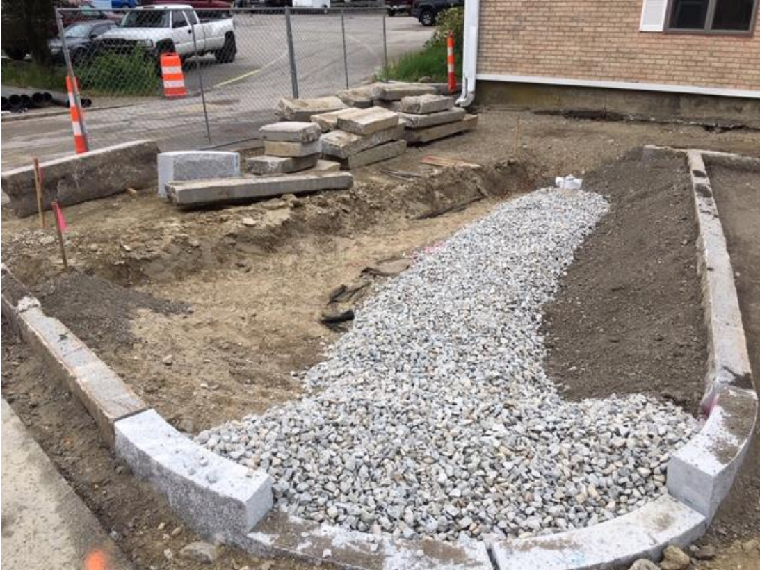
South Main Street – Rain Garden South of Municipal Parking Lot
