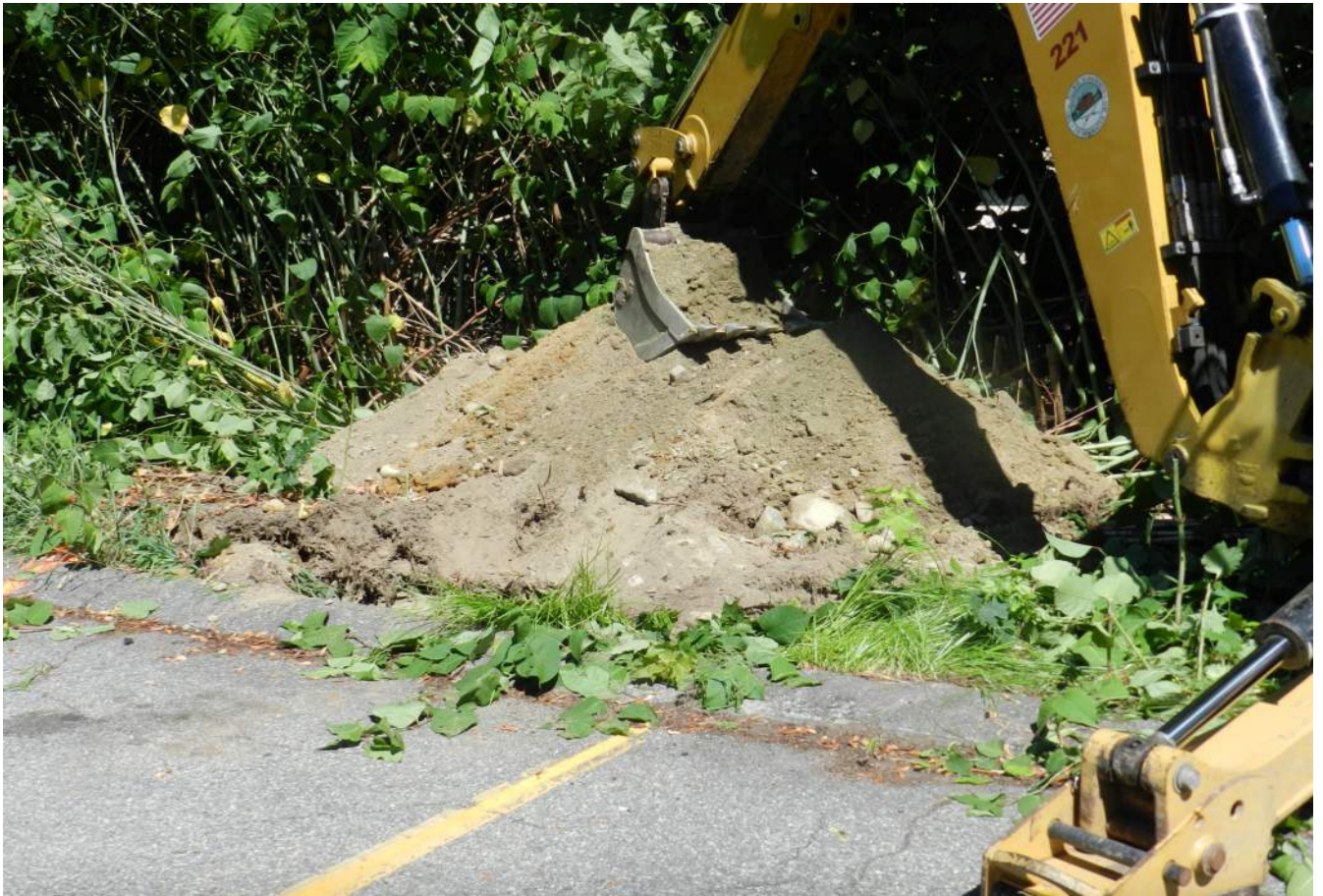
Test Pit 3. - Excavation Stockpile.
