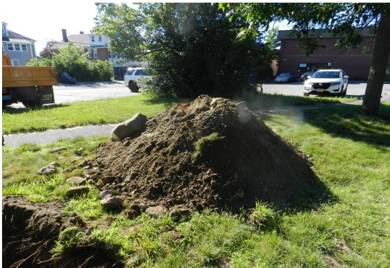
Test Pit 2 - Excavation Stockpile
