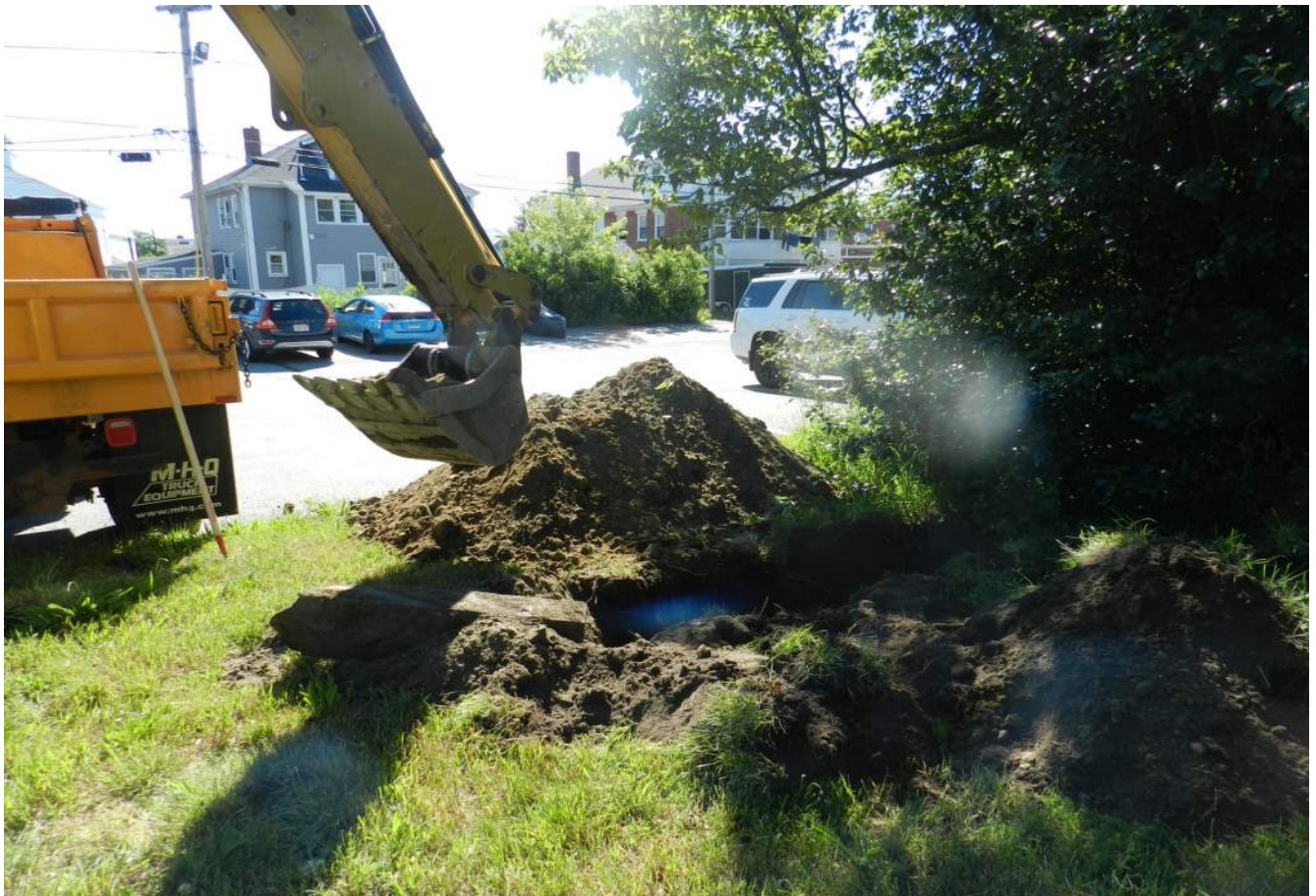
Test Pit 4 - Excavation Stockpile.
