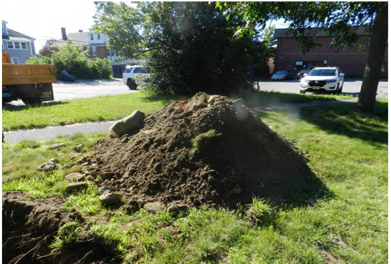
Test Pit 2 - Excavation Stockpile
