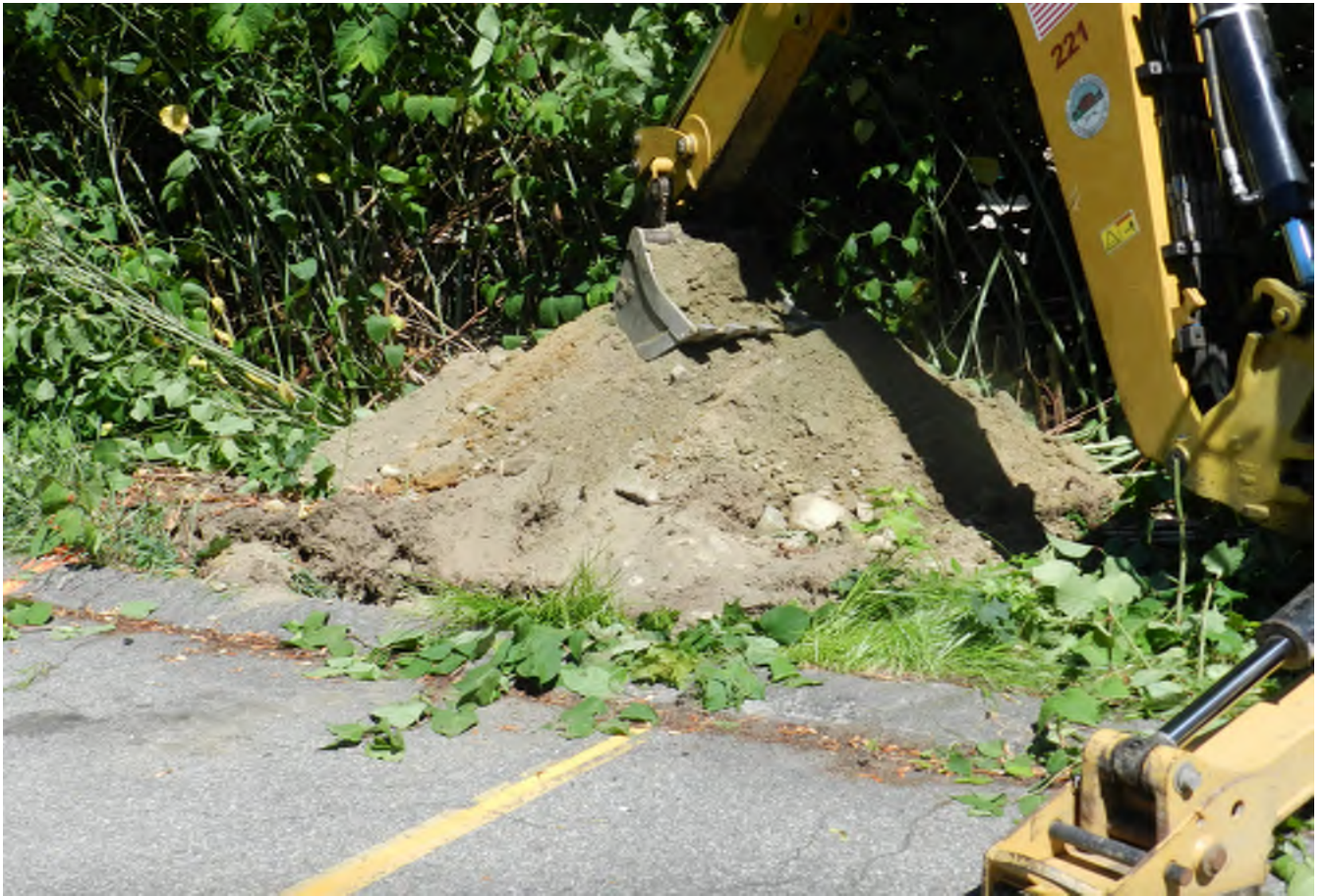
Test Pit 3. - Excavation Stockpile.
