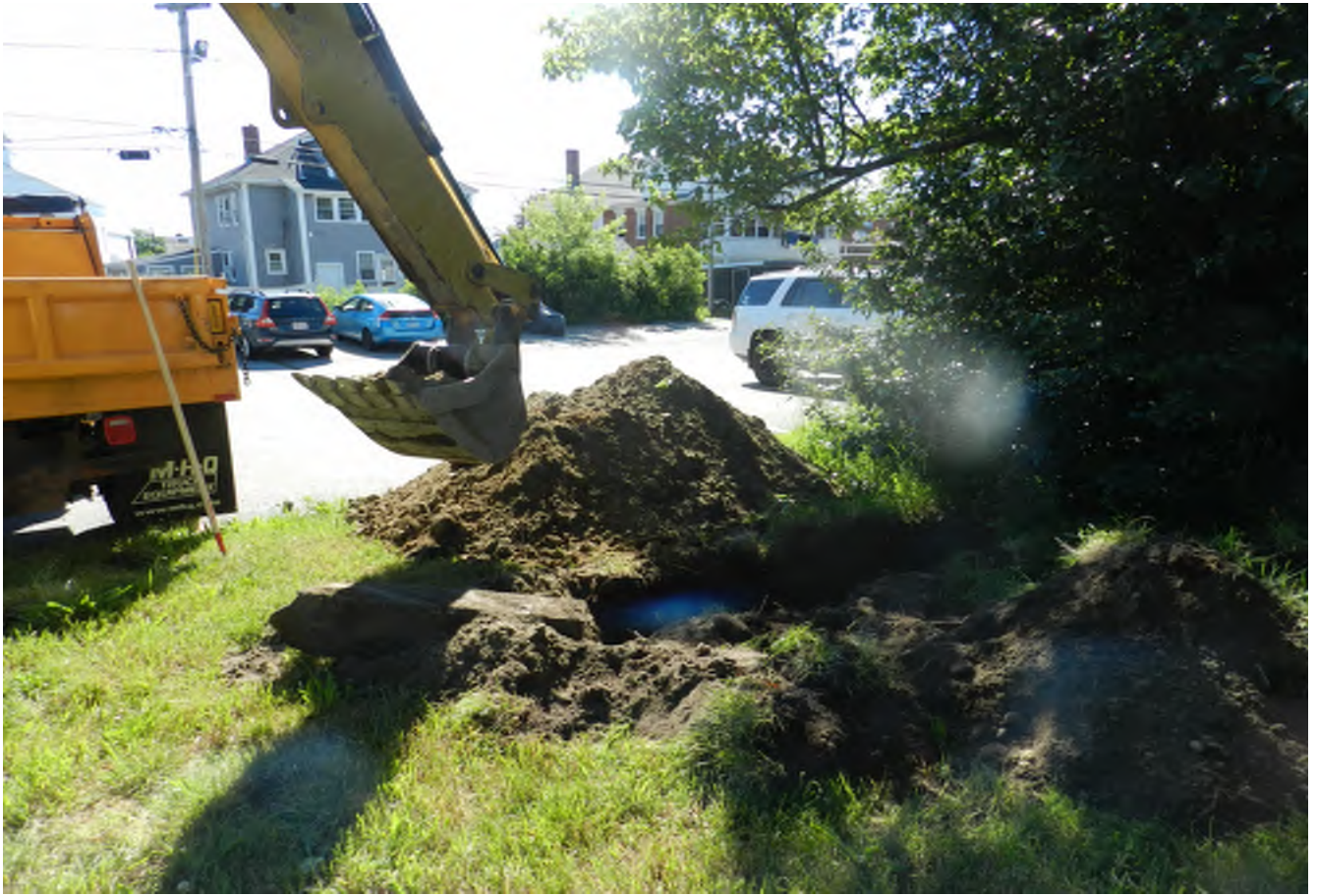
Test Pit 4 - Excavation Stockpile.
