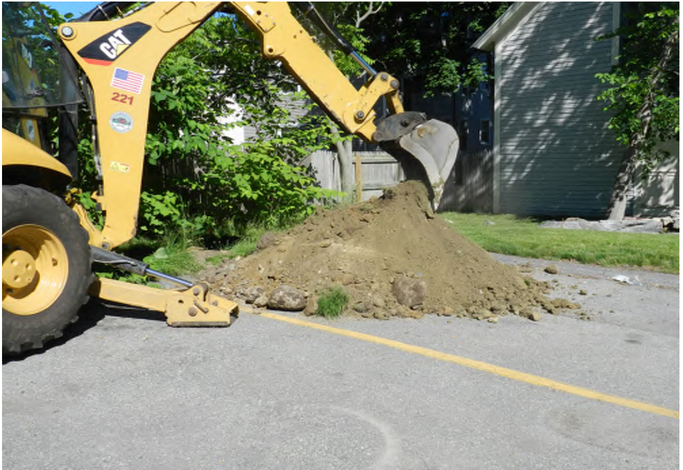
Test Pit 1 - Excavated soil pile
