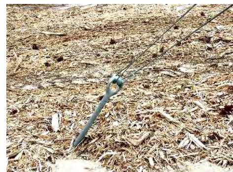
An anchor, installed, with 2 guy wires attached
