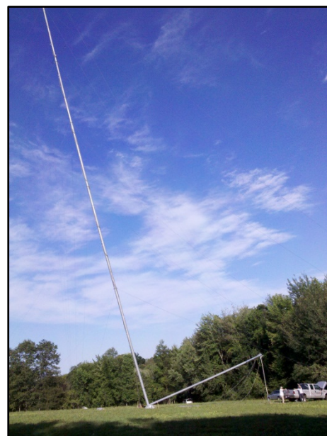
Photo 3 – MET Tower Installation
